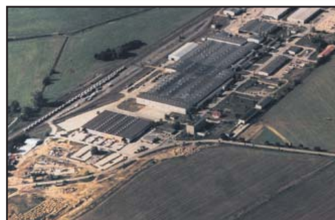
Holzwerke Bullinger Production Facility in Neuruppin, Germany.
