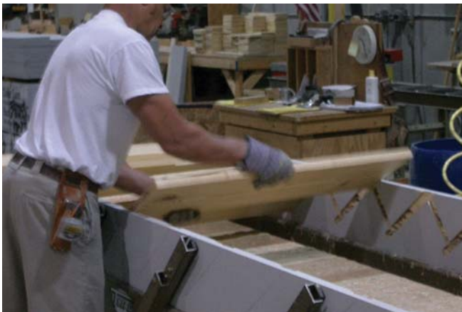
Placing treads (steps) inside stringer grooves
