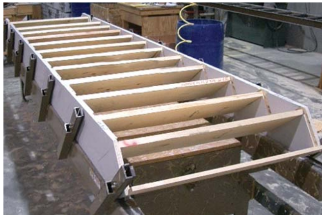
Master Stair stair steps completed
